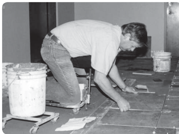
Solution: Laying tile with kneeling creeper
