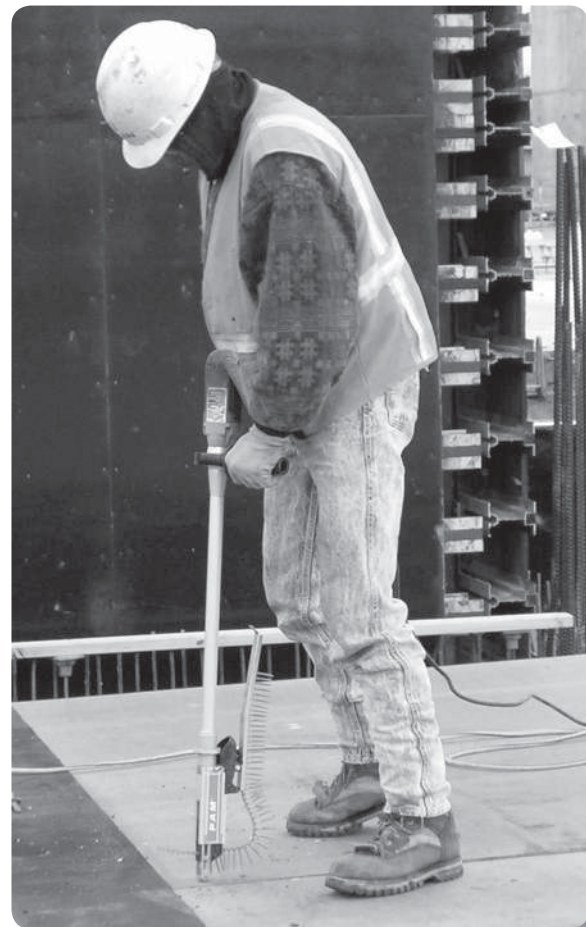
Solution: Autofeed stand-up screw gun
