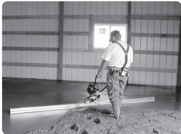
Solution: Motorized screeding
