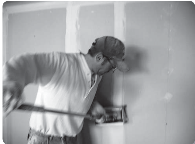
Problem: Hand drywall finishing with mudbox
