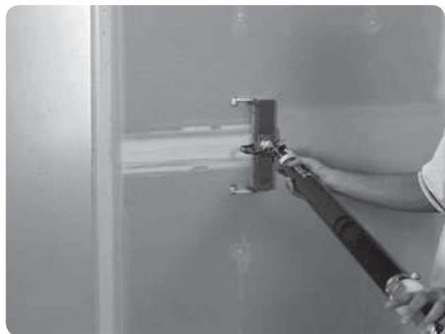
Solution: Pneumatic finishing system
