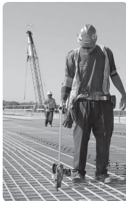
Solution: Rebar-tying tool with extension handle
