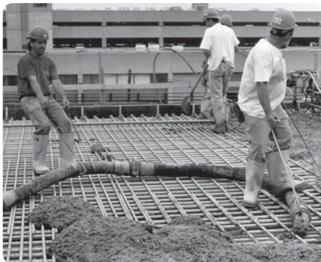
Problem: Pulling concrete hose without skid plate
