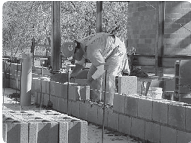
Problem: Laying standard concrete block
