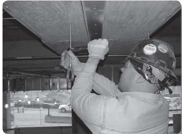
Problem: Tightening conventional nut on all-thread
