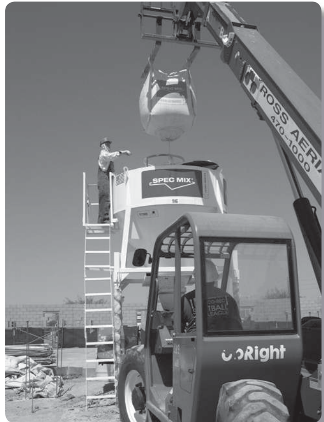
Solution: Loading a silo system
