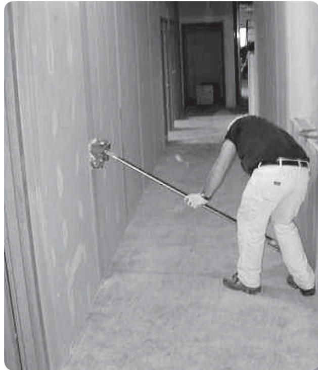
Problem: Hand drywall finishing with mudbox
