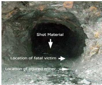
Victim was struck by blast debris that traveled through a diamond core hole.
