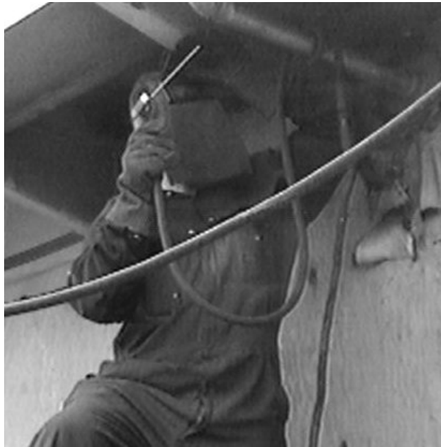
Figure 12. Shipboard Pipe Welding
