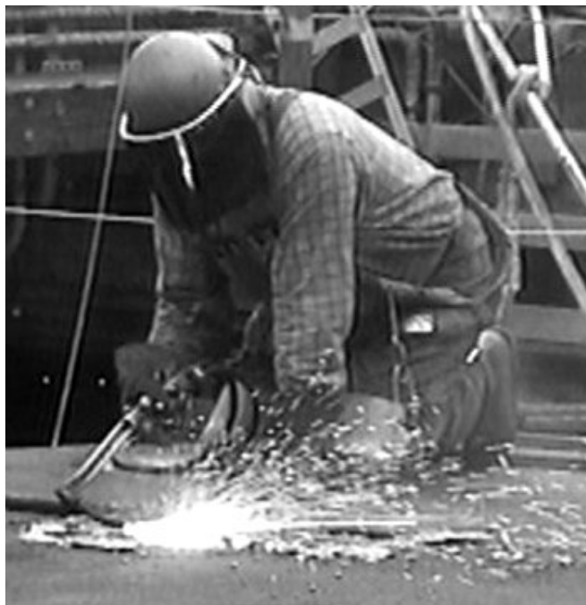
Figure 28. Torch Cutting Deck
