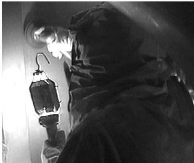
Figure 26. Shipboard Tank Grinding
