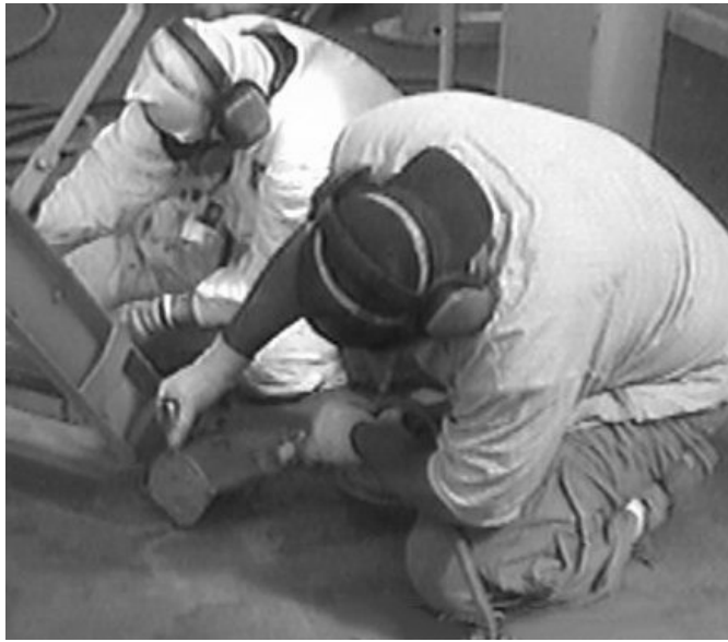
Figure 27. Deck Scraping
