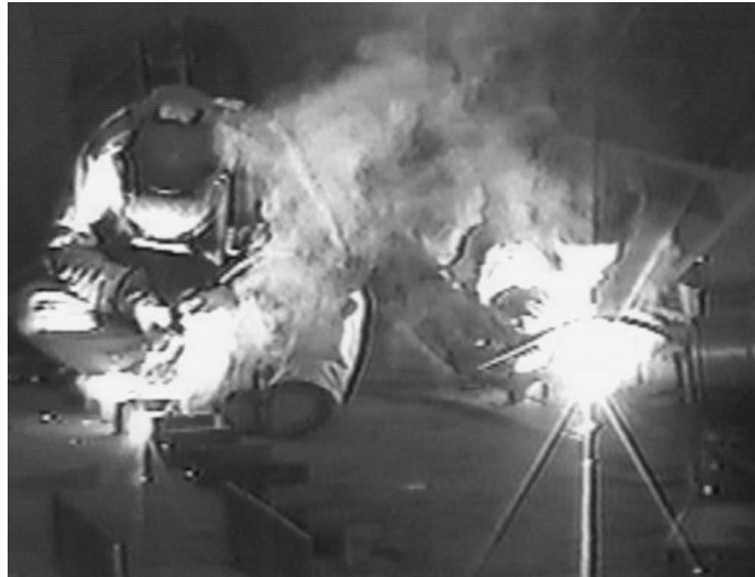
Figure 19. Engine Room Welding
