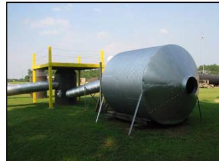
A deck has been built over one of the manholes to allow for an elevated vertical entry point. Consideration should be given to construction a second deck with an offset hole and converging walls to provide a higher degree of difficulty for more advanced members.
