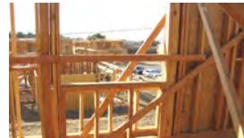
**Ladder openings** need to be guarded with off-set guardrails or swinging gate must be provided.
