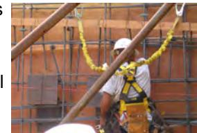
**Note:** Point to point travel on rebar is allowed without fall protection for heights up to 24 feet.
