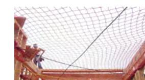
**Floor covers** need to be provided for all floor openings, hatchways, floor holes, and skylight openings regardless of the fall heights. Floor openings can be alternatively guarded by guardrails.
