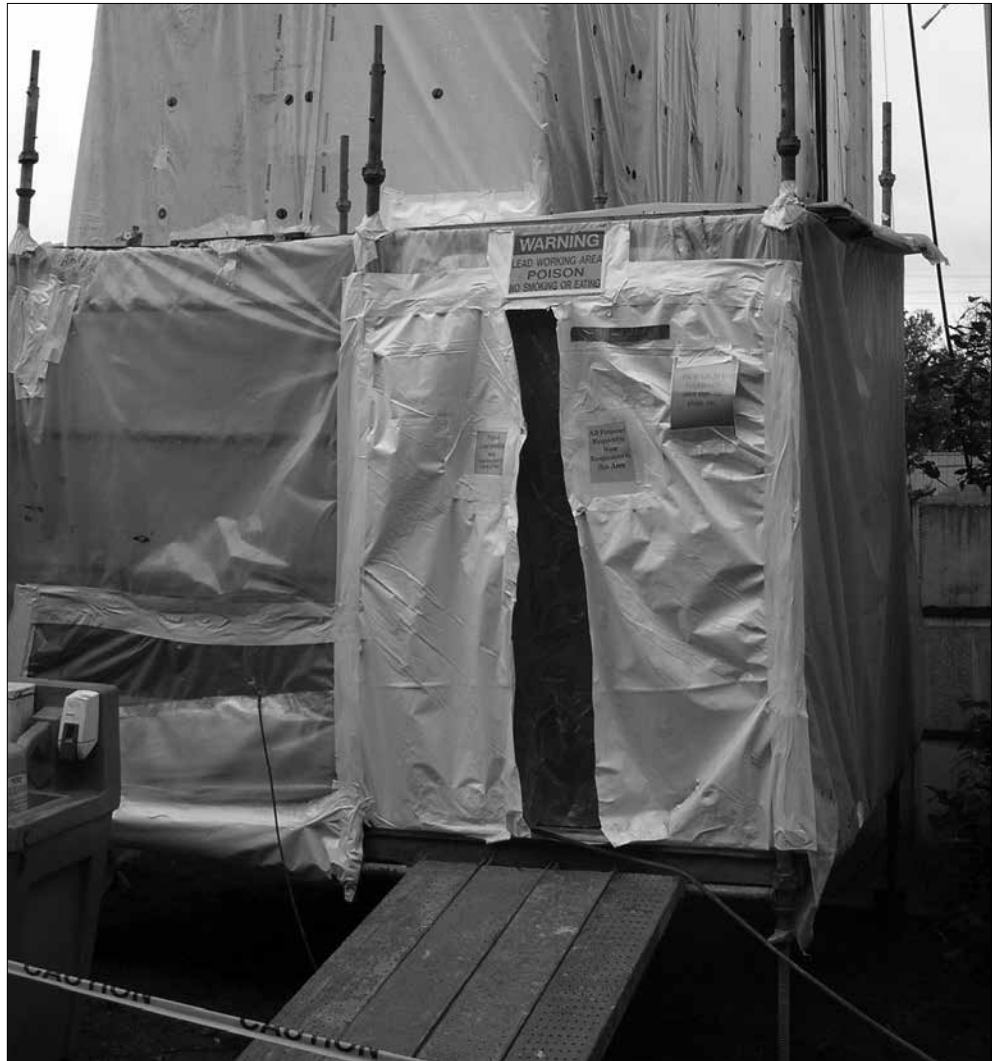
Entrance enclosure for lead removal
