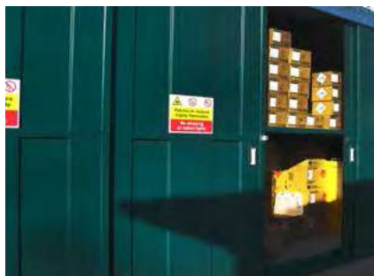
Advanced storage of chemicals in different safety compartments
