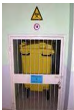
Interim waste storage ready for collection
