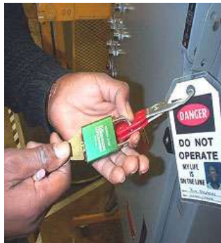
Locked out electrical box
