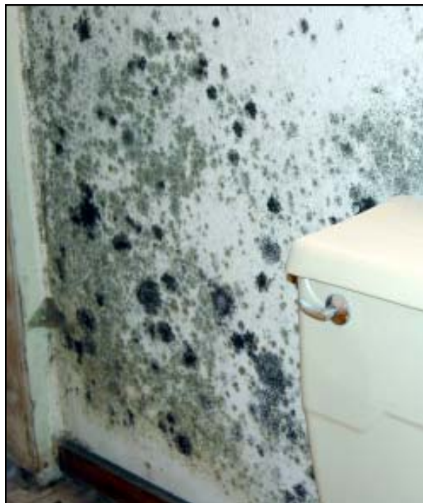
Many mold colonies growing on dry wall in a residence. (Image courtesy of Dr. Chin S. Yang of P&K Microbiology Services)
