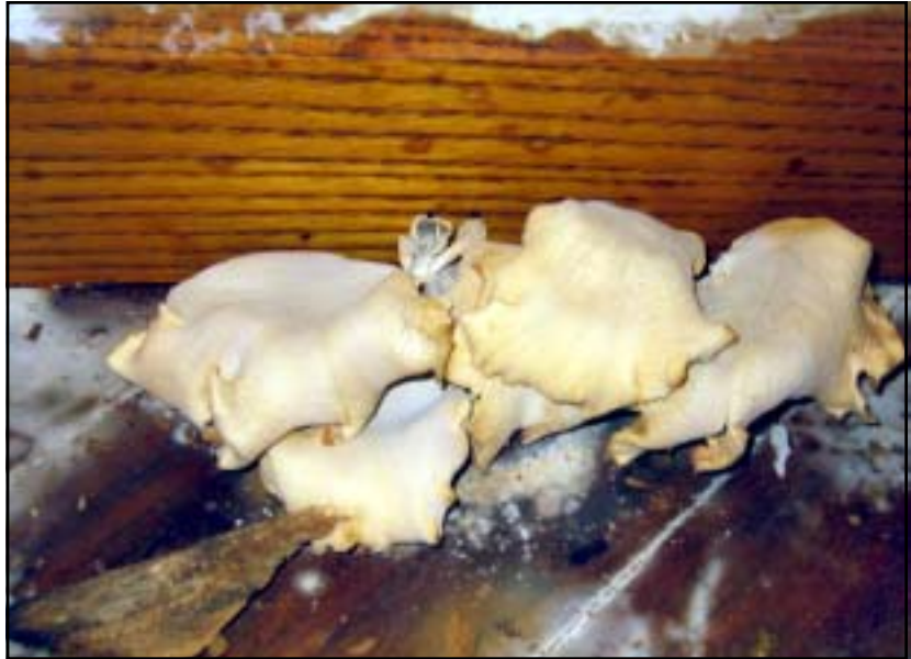
Mushrooms produced on hardwood floor where there has been long-term water incursion. (Unknown or anonymous author. Image courtesy of Dr. Chin S. Yang of P&K Microbiology Services)
